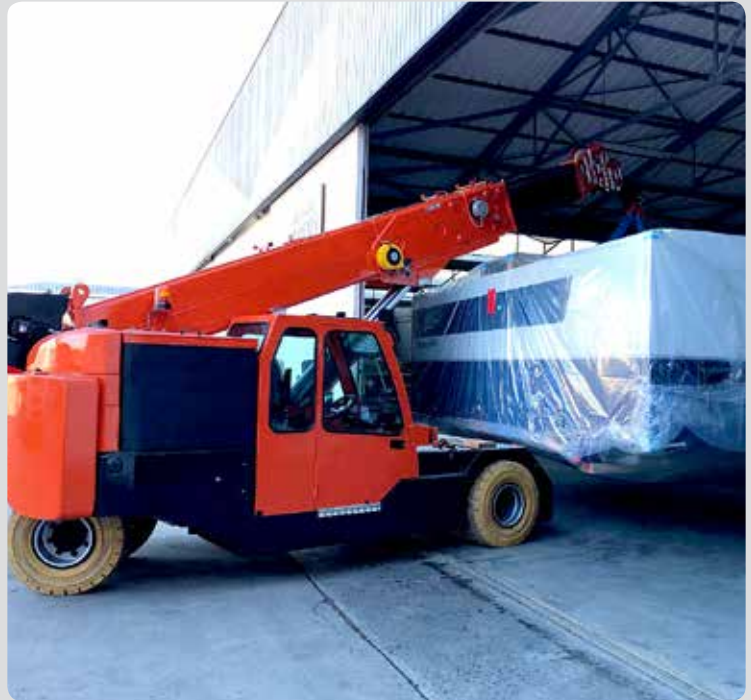
GF250 Pick & Carry Crane lifting with a rhino hook (Capacity: 16800kg).
