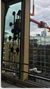
Libro 2500B fitted with a modified MRTA8 vacuum lifter on a manipulating head for installing GRC soffit panels
