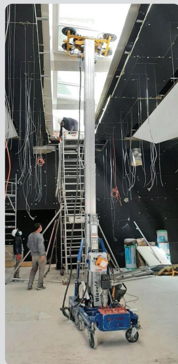
The GML500+ can also be used with its own optional glass vacuum lifter with radio remote for total control when glazing at height. The maximum capacity is reduced if using the VGL98 Glass Vacuum Lifter to 350kg.
